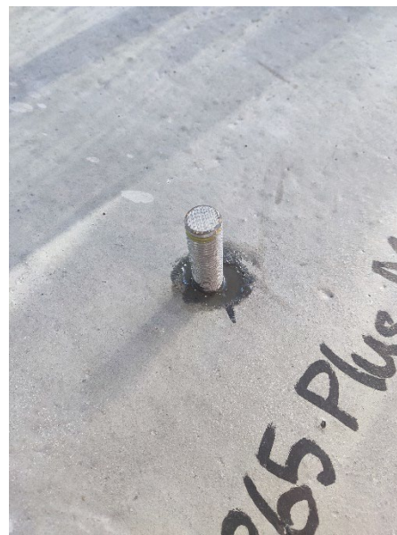
b) Anchor installed with EP65 PLUS epoxy
