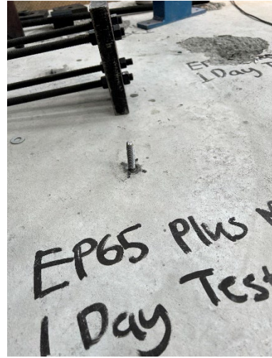
f) Anchor installed in concrete
