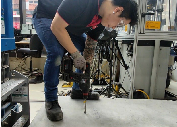
a) Drilling of hole
