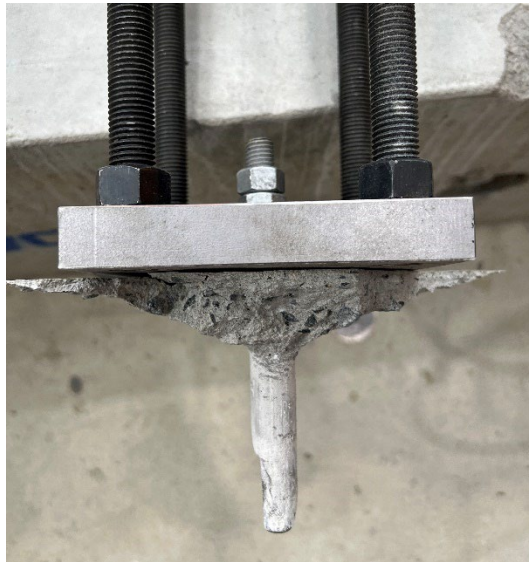
c) Mixed mode failure
