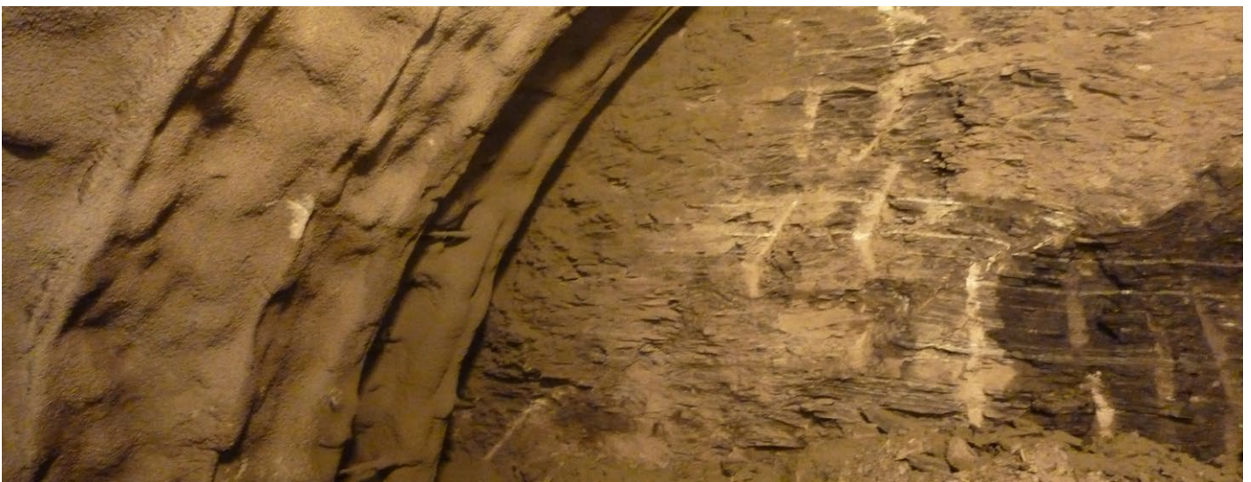
Drill & Blast Method
