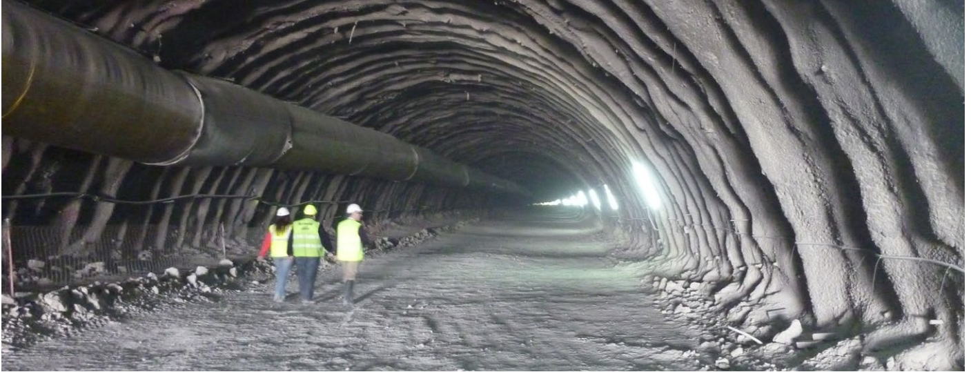
New Austrian Tunneling Method (NATM)
