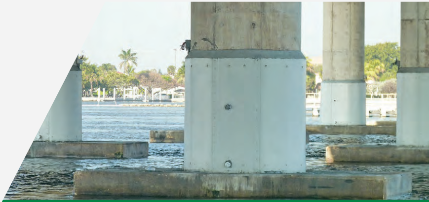
Galvashield® DAS Jackets Installed
